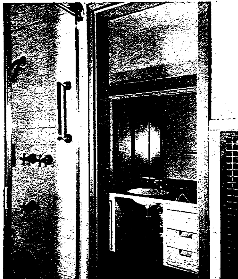
Only a bathtub and shower are located in the bathroom, while in area next to it are lavatory and dressing room.
