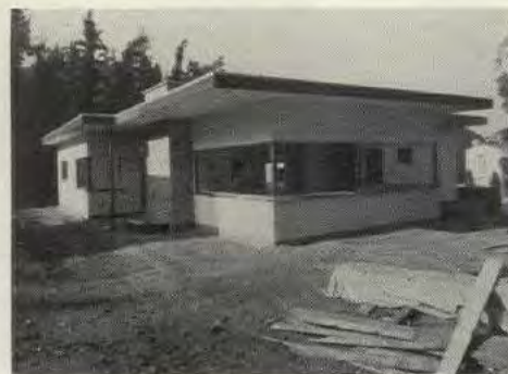
LOW COST HOUSE, built by Ban in Los Angeles, uses the columns he designed for economy and to open long, unbroken stretches of window area in living room.
