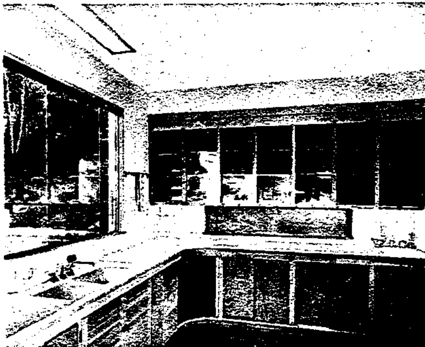
Sliding windows of plate glass are featured throughout the house. In the kitchen they are utilized behind the sink.
